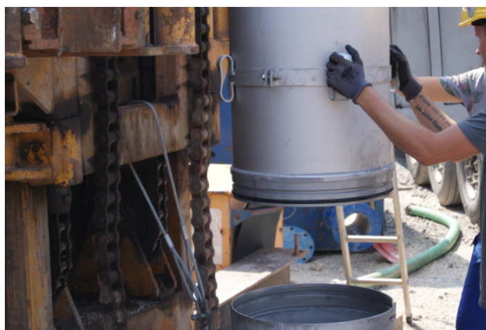
Picture 1: Installation of DN500 casing with ZSM connection
